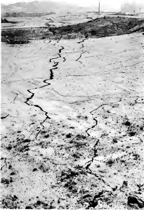
Photo 13. Ground cracks resulting from lurching. Courtesy of H. G. Anderson, Los Angeles Valley College.
